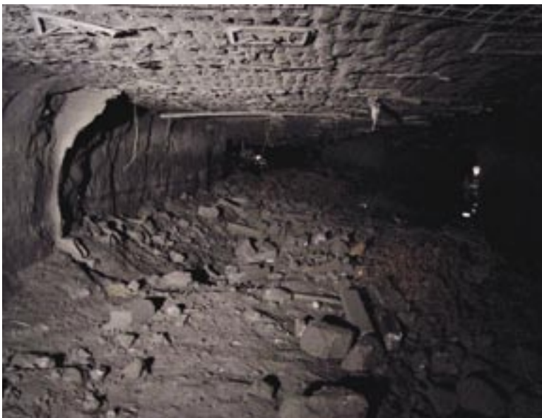
Area inby the Omega Block seals after the explosion. Debris is scattered over the entire area and a thick layer of soot covers everything.
