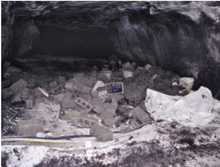
The remains of a concrete block wall after being struck by the forces of the explosion. It is still possible to see some of the blocks strewn around the area.
