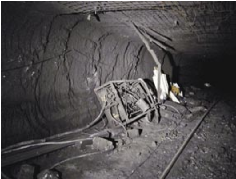
Damaged charging station located in the mains outby the sealed area.
