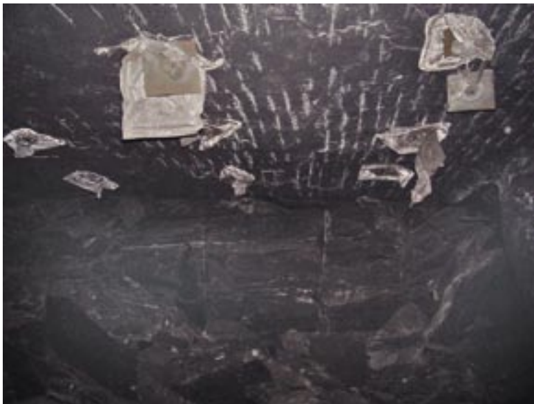
Damage to the roof supports (pie pans, roof bolts and plates) from the forces of the explosion. There is a roof fall in the foreground.
