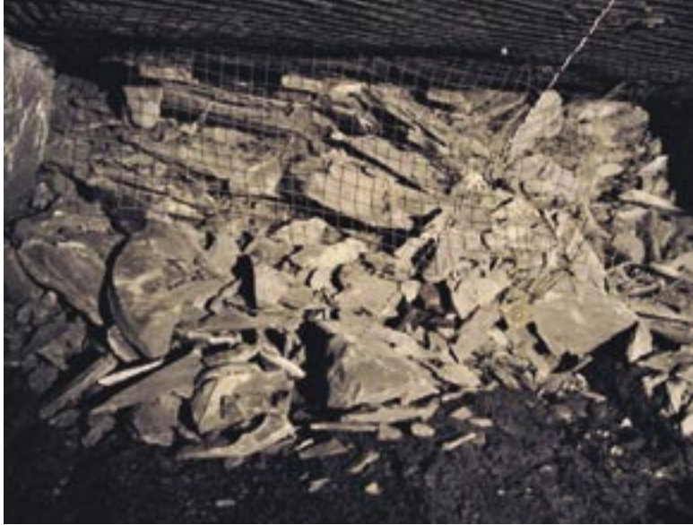
Roof falls are a hazard in the mining industry. The picture to the left was taken in the 2 nd North Mains Section after the explosion. The investigation revealed numerous falls in the area that had occurred after it was sealed. Roof fall have been documented to cause frictional arcing.
