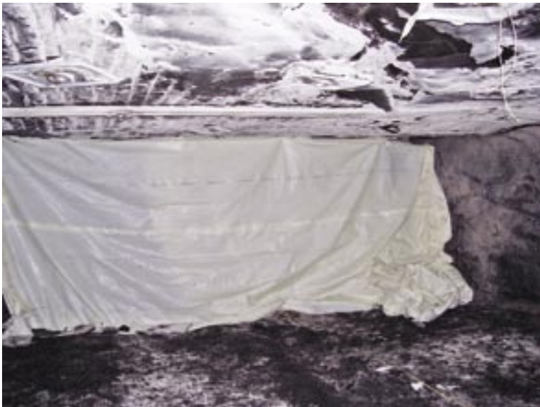
Outby view of the barricade constructed by the 2 nd Left crew in an attempt to isolate themselves from the contaminated mine atmosphere.
