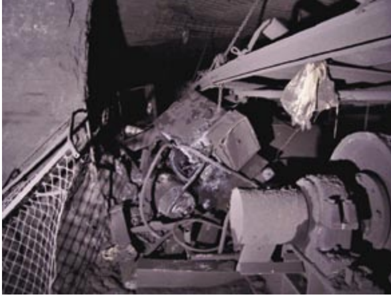
Damaged 2 nd Left belt drive. The drive was located at 58 block, approximately the location where the miners were forced to abandon their first rescue attempt.
