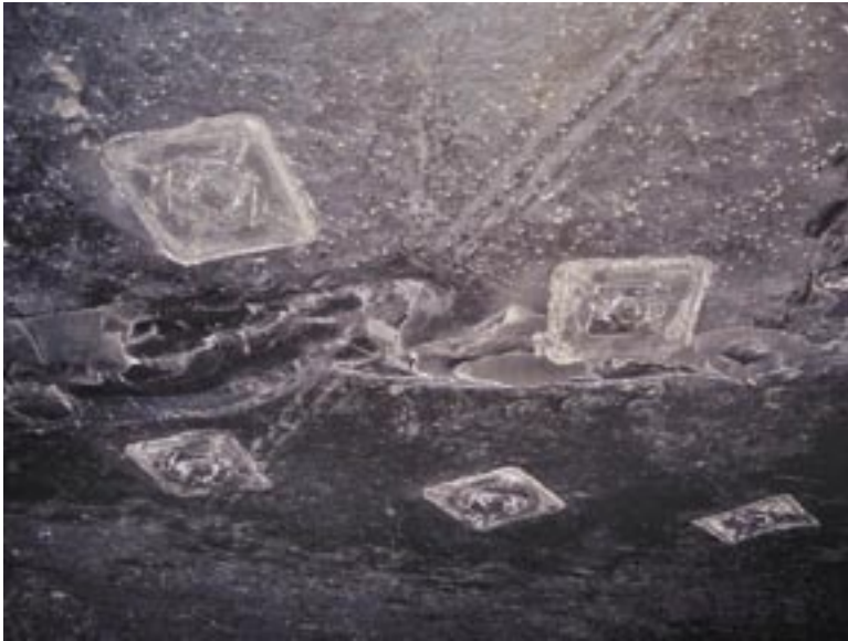
During the investigation the marks in the roof pictured at the left drew much attention. The "anomaly," as it became known, was later determined to be a fossil.
