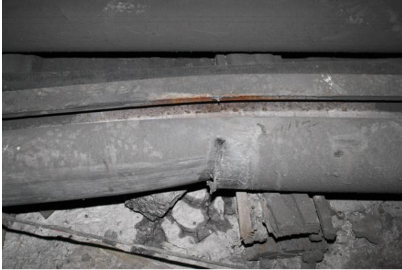
Figure 9). (LEFT) Bent track and punctured waterline, at location “B” (see the figures below).
