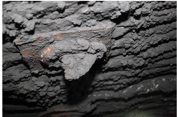
Figure 4A. (LEFT) Impacted “mud” on east side of header board across entry #2, between BRK 32 and 33, and about 70 feet inby spad 22806.
