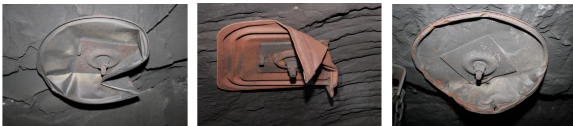
Figure 8. (Left) An example of a roof pan Not Rusted Figure 9. (Middle) An example a roof pan Mostly or Entirely Rusted. Figure10. (Right) An example of a roof pan with Edges, Only Rusted
