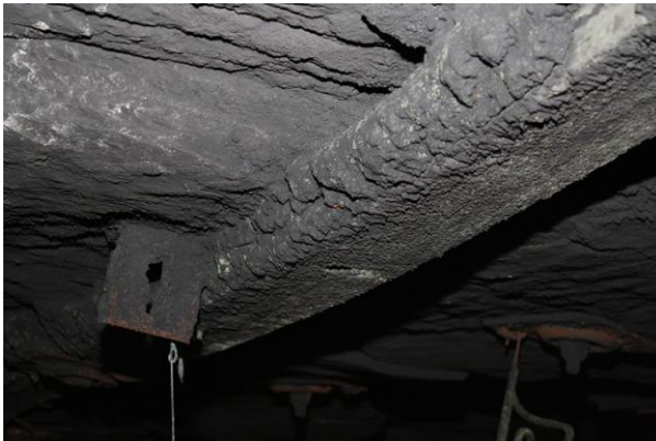
Figure 4A. (LEFT) Impacted “mud” on east side of header board across entry #2, between BRK 32 and 33, and about 70 feet inby spad 22806.
