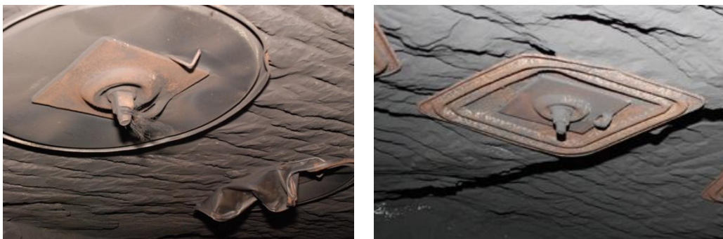
Figure 1. (LEFT) Example of round pan (pizza pan). (RIGHT) Example of square pan (spider plate).
