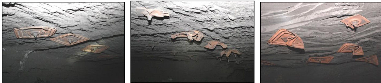
Figure 5. (Left) An example of “NO PAN BENDING.” Pans bent < 90 degrees.
