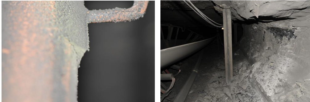
Figure 12. (LEFT) Sand jack with dust cone (lower part has fallen away); #21 Tailgate, approximately 2 breaks east of the Longwall, looking North. Final Forces were from the EAST
