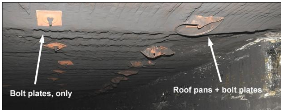
Figure 2. Example of roof pans (right) after explosion. Typically, four lines of bolts are installed on 4-ft. centers, but only one line incorporates roof pans at UBB. Additional roof pans are installed as roof conditions require. Round pans or “pizza pans” are used in this example.
