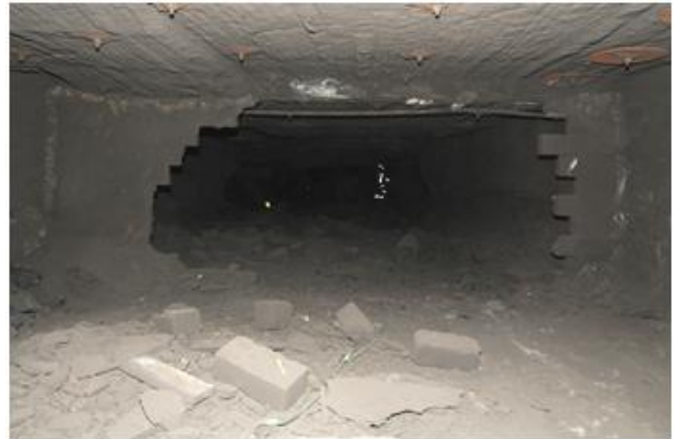
Figure 4. (LEFT) Concrete block stopping, with a remainder pallet of unused block.
