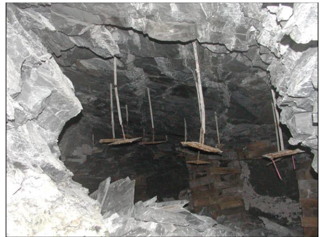
Figure 16. An example of coal mine shale roof unraveling between roof bolts in response to internal strains and reduction in rock strength caused by moisture adsorption.
