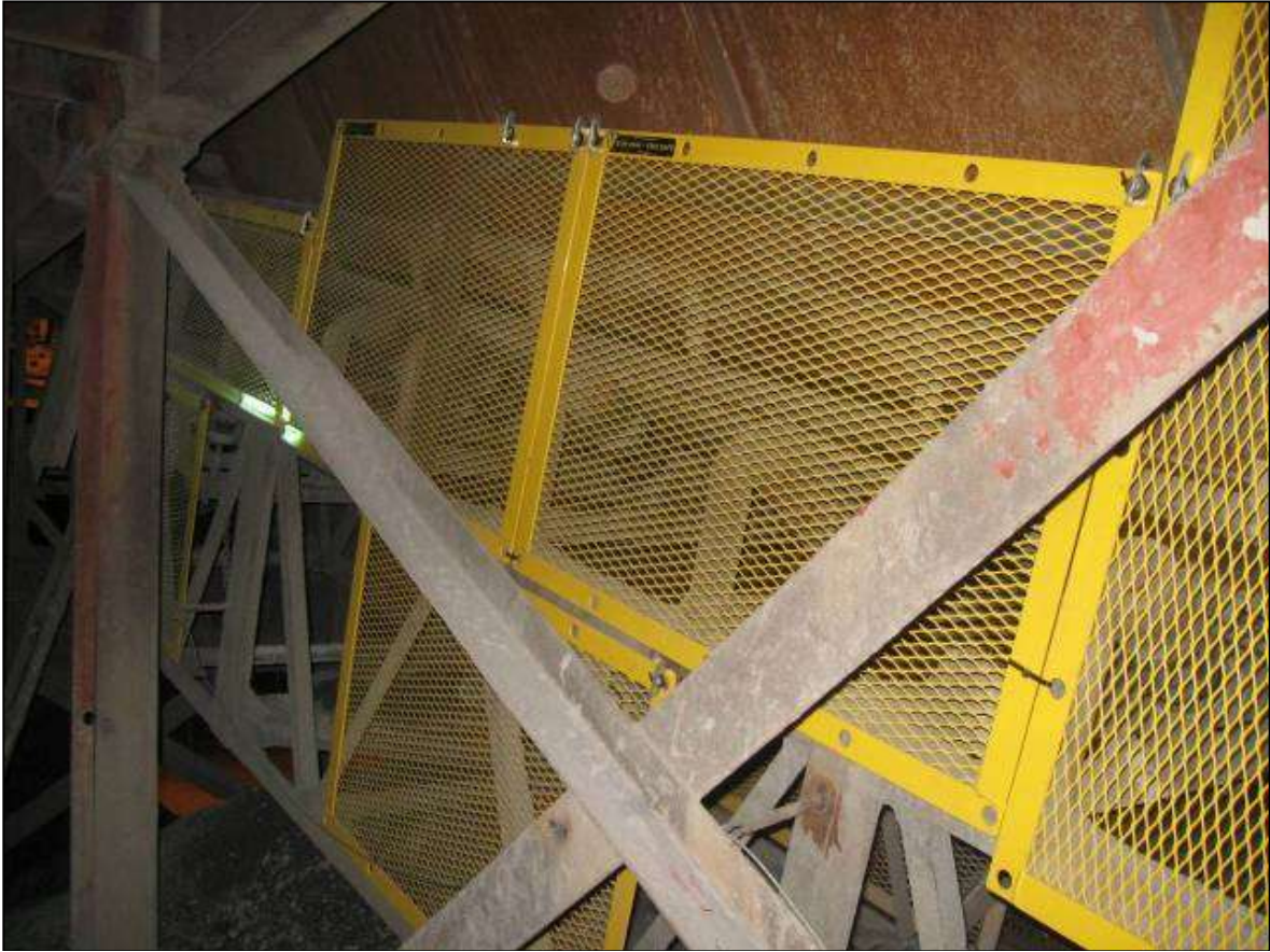
Receiving Hopper/Skirt Boards
