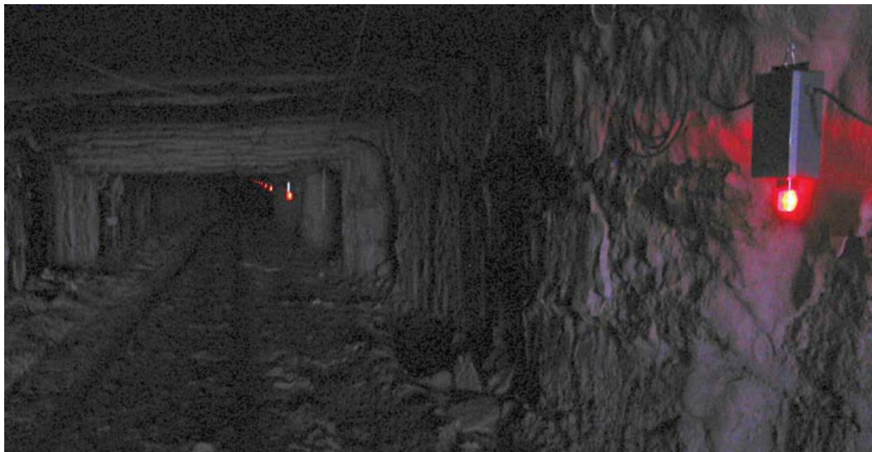
Figure 104 – Typical Installation of the MineTracer System from Venture Design Services
