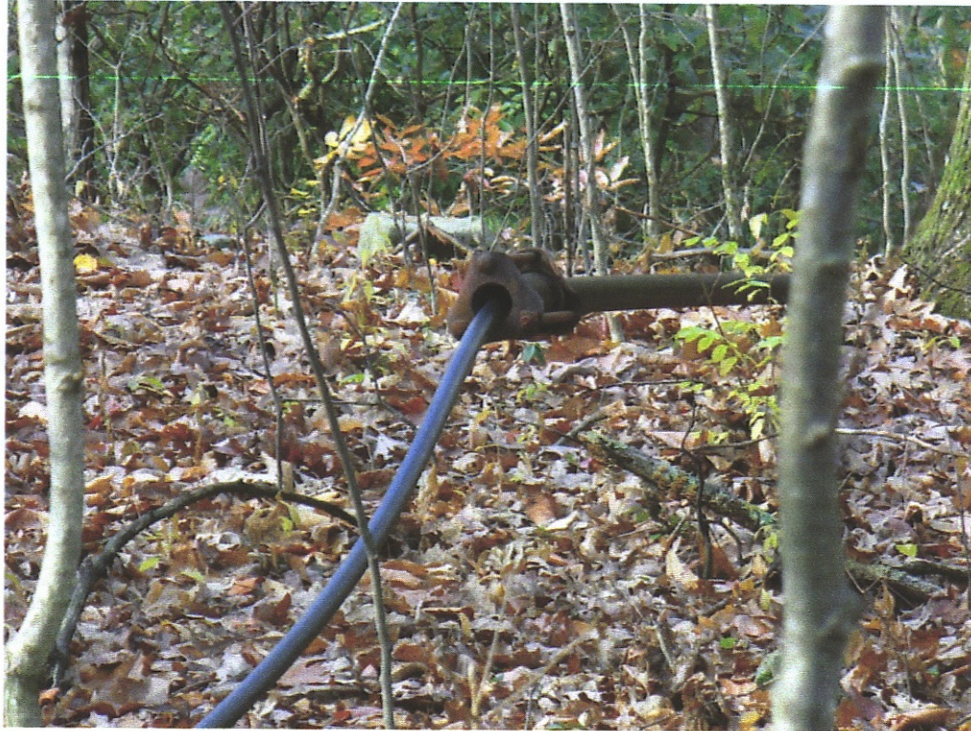
Photo 2: A Twenty Five Foot Break In Trubie Run Steel Gas Line And Spliced Together With Plastic Gas Line
