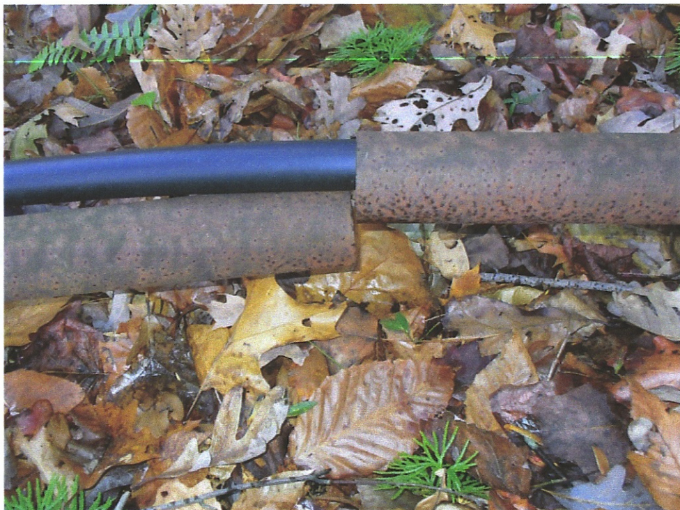
Photo 4: Break In Trubie Run Gas Line And Spliced With Plastic Gas Line
