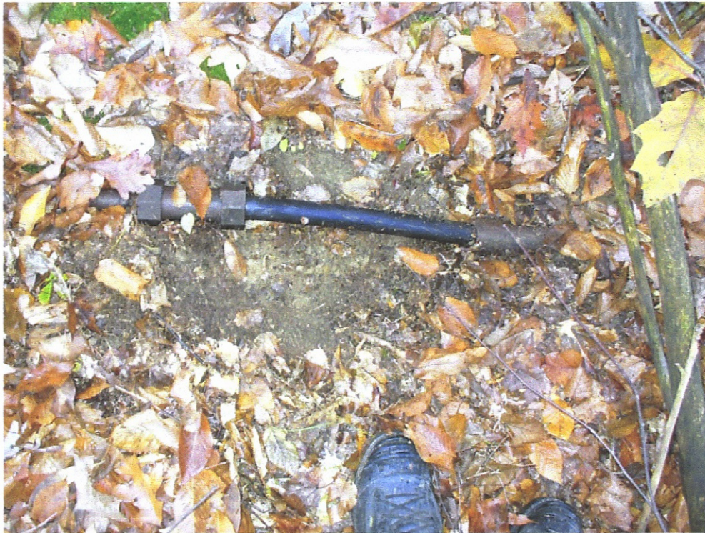
Photo 3: A Two Foot Break In Trubie Run Gas Line And Spliced With Plastic Gas Line
